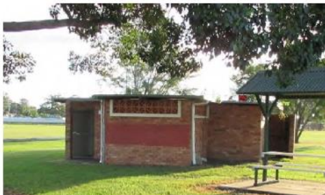
Disconnected amenities building near athletics oval
