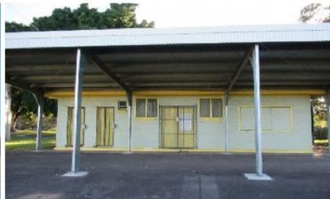
Cricket club house building & canteen
